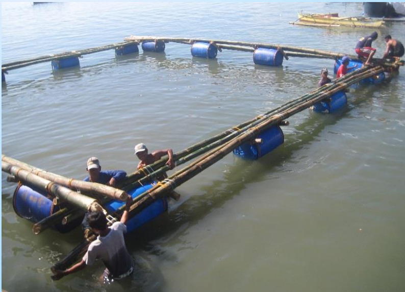
Fabrication of cage frame
