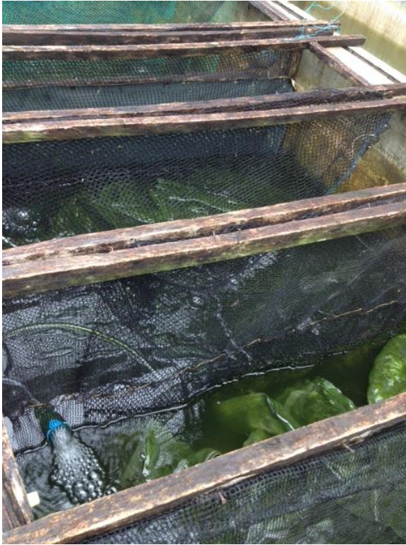
View of net substrate in biofilter
