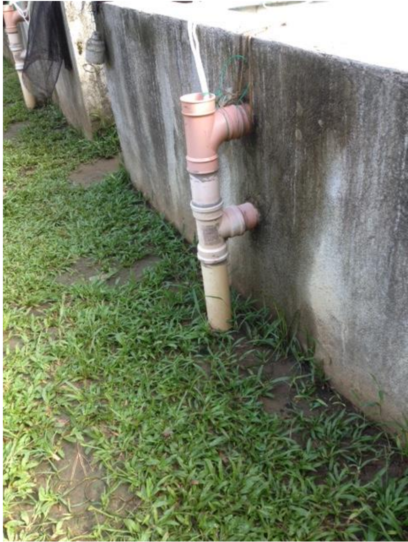
Airlift pump at inlet of tank
