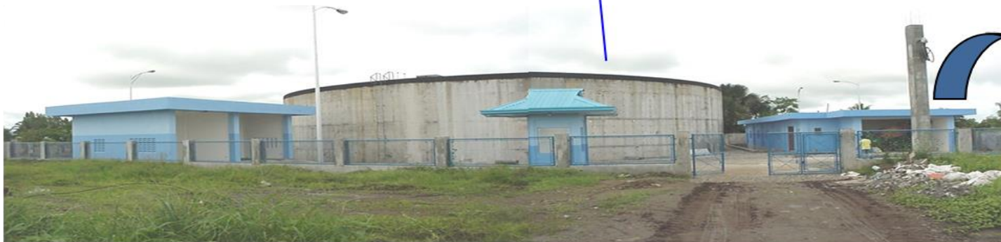
6,500 cu.m. Ground Reservoir w/ Booster Station
