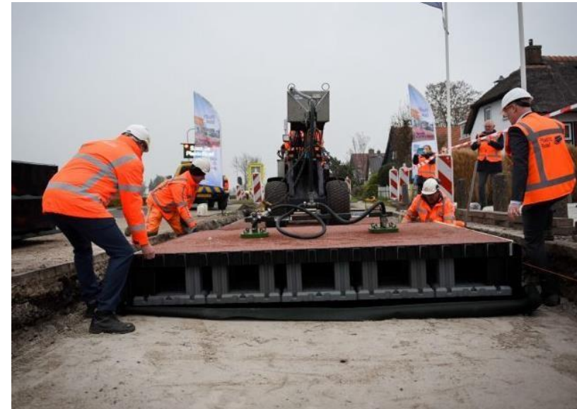
Construction of 2nd PlasticRoad bicycle path in Overijssel, Netherlands, Nov 22, 2018
