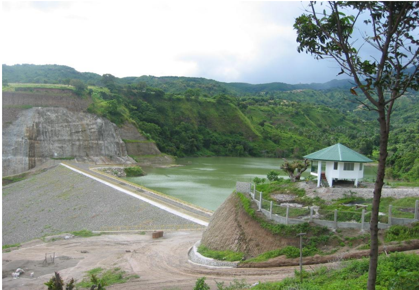
Impounding Earthfill Dam
