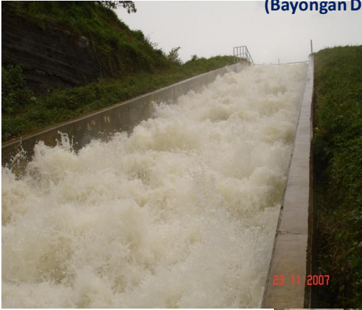
Diversion Chute – conveys water from Malinao Dam to Bayongan Dam
