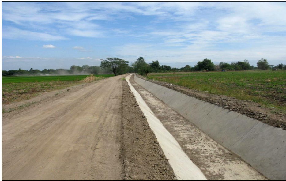
Lateral Canal with Service Road in the Mt. Pinatubo-affected TARRIS Service Area
