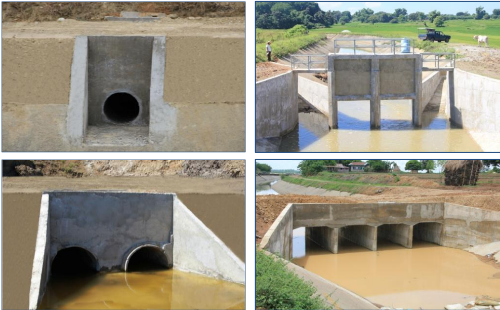
Some of the Completed Structures in the North Main Canal Area
