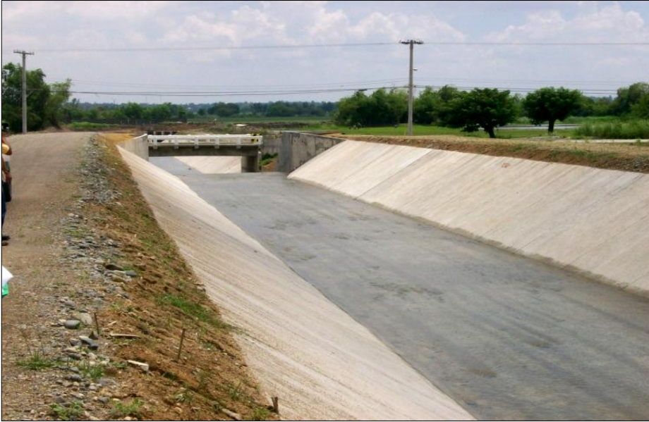
Two-Lane Bridge with a Drop Structure at North Main Canal
