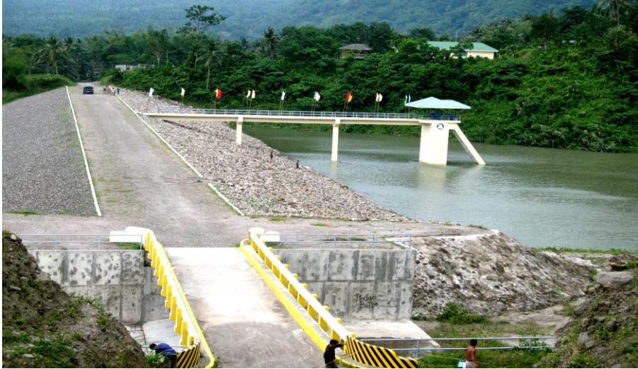
Impounding Earthfill Dam
