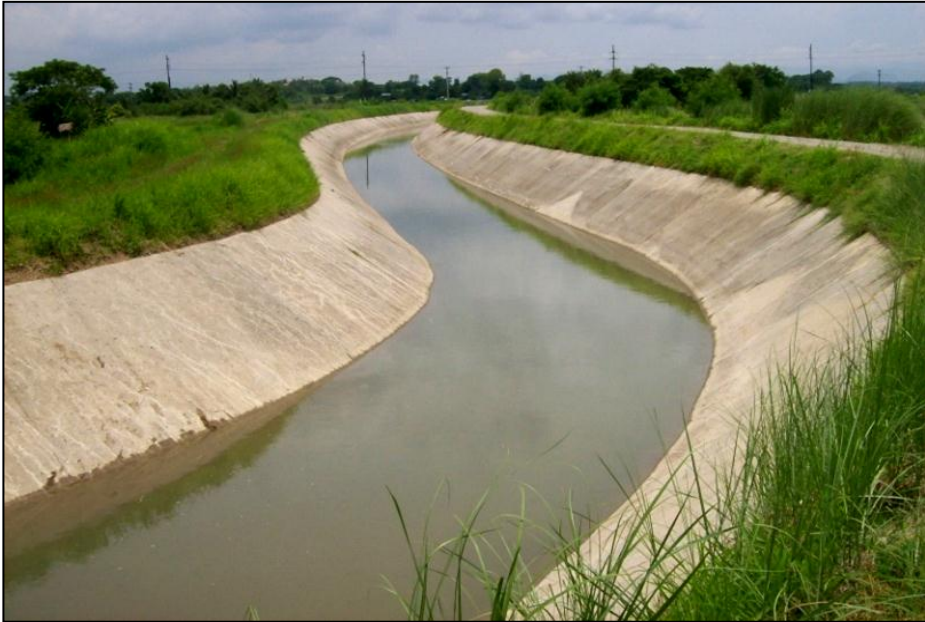
Upstream Portion of North Main Canal
