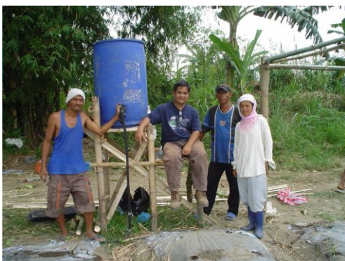
Installation of gravity drip irrigation in Maguindanao and Sultan Kudarat
