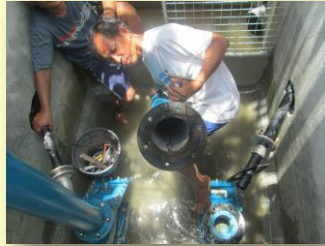
Installation of ram pump
