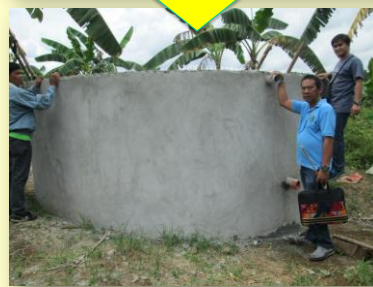
Construction of ferro-cement reservoir
