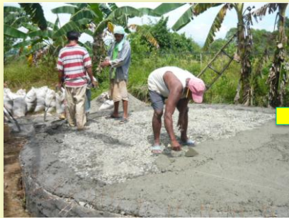
Construction of ferro-cement reservoir
