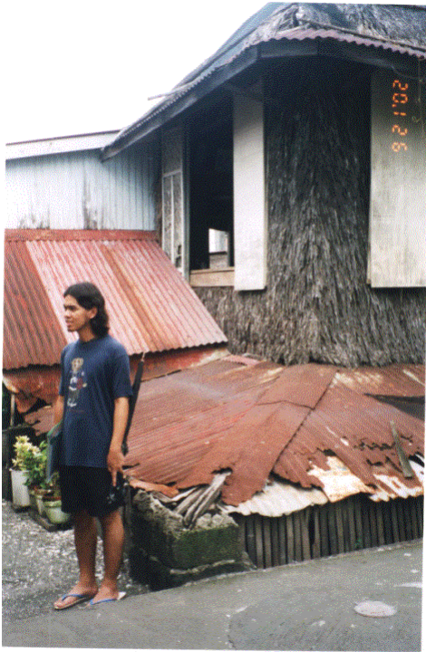
Slowly buried house, Bgy. Binaungan, Obando, Bulacan
