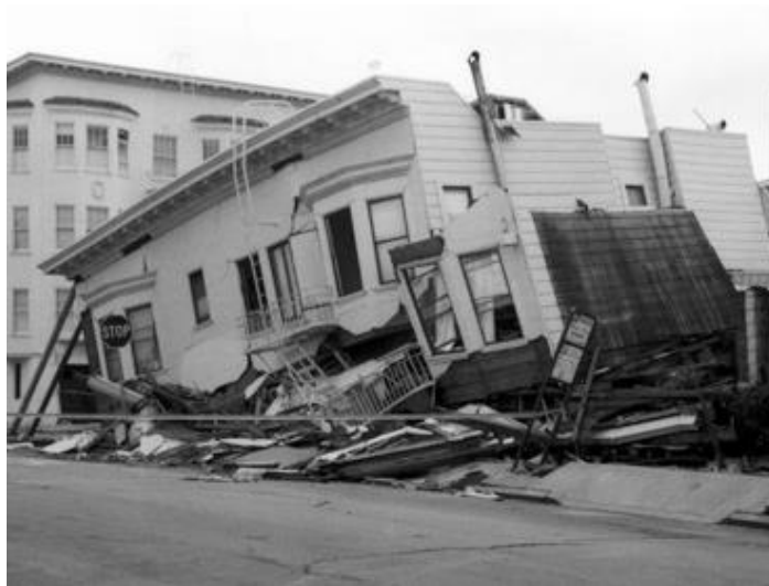
Liquefaction in the Marine District in San Francisco, Calif., caused damage during the October 1989 Loma Prieta earthquake.
