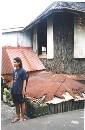
Slowly buried house, Bgy. Binaungan, Obando, Bulacan - F. Siringan, UPMSI
